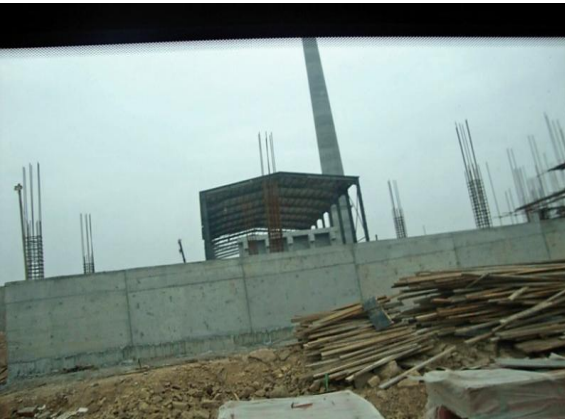
Coal storage unit
